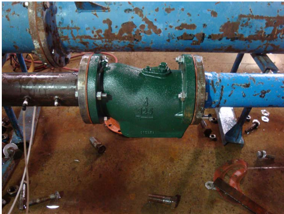
Figure 1. 4-inch strainer installation (Metraflex strainer shown).
