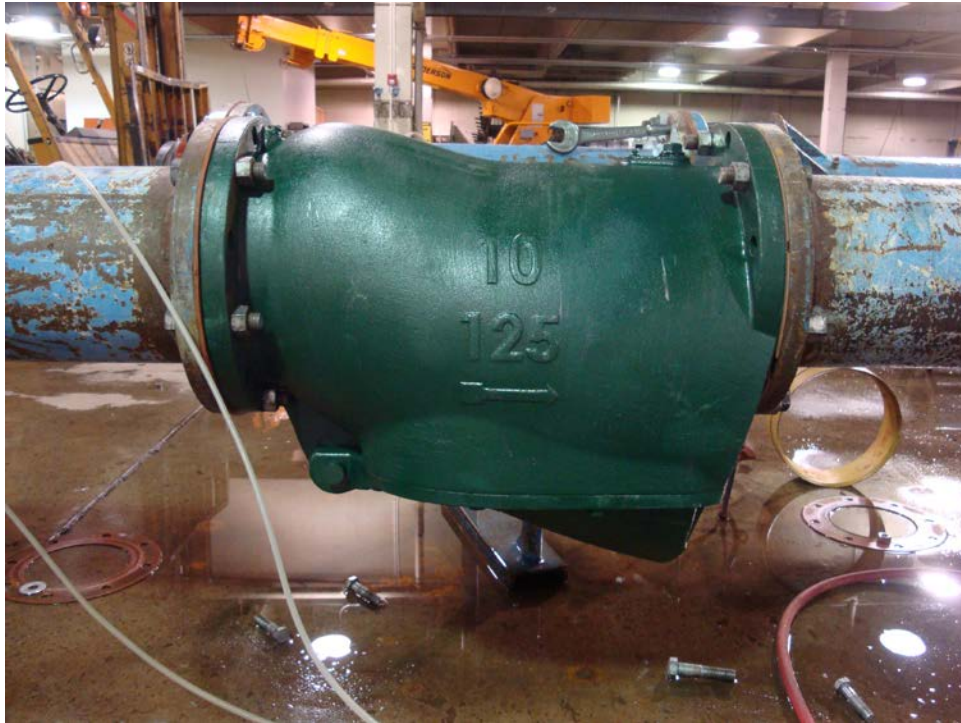
Figure 3. 10-inch strainer installation (Metraflex strainer shown).
