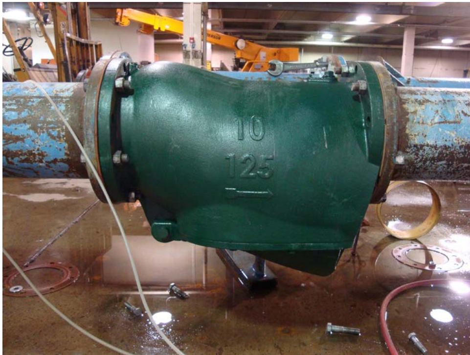
Figure 3. 10-inch strainer installation (Metraflex strainer shown).
