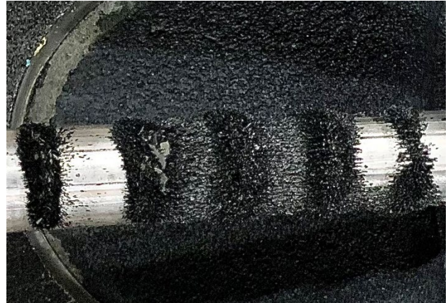
Figure 1 The LPD Mag cover plate and attracted particulates shown before the blow down of the second LPD Mag Y Strainer
