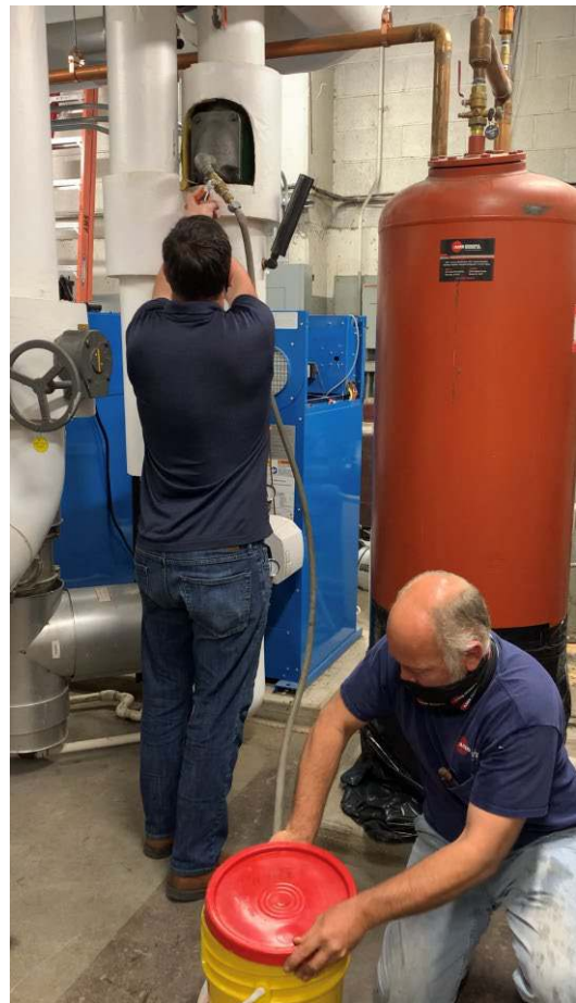
Figure 1 The LPD Mag cover plate and attracted particulates shown before the blow down of the second LPD Mag Y Strainer
