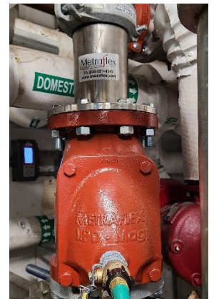
Figure 2 LPD Mag Y Strainer with Spool Piece
